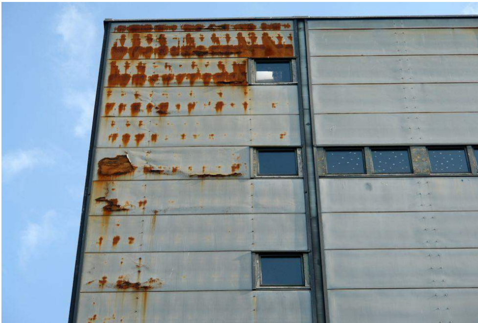
Figure 8. The intense blue of the façade was completely withered away, showing rust in many places
