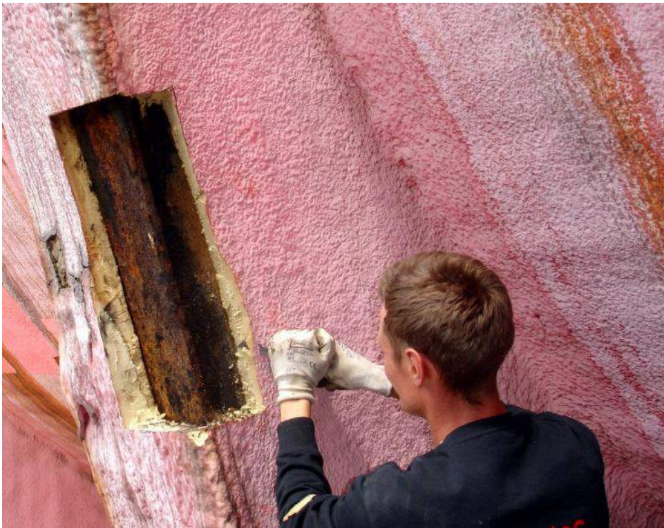
Figure 11. Dutchmen's repair for PU foam
