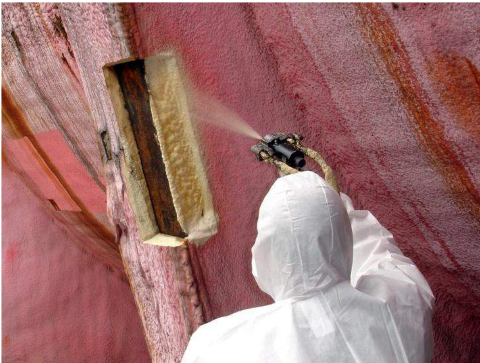
Figure 12. Filling of the square cut outs with "new" PU foam
