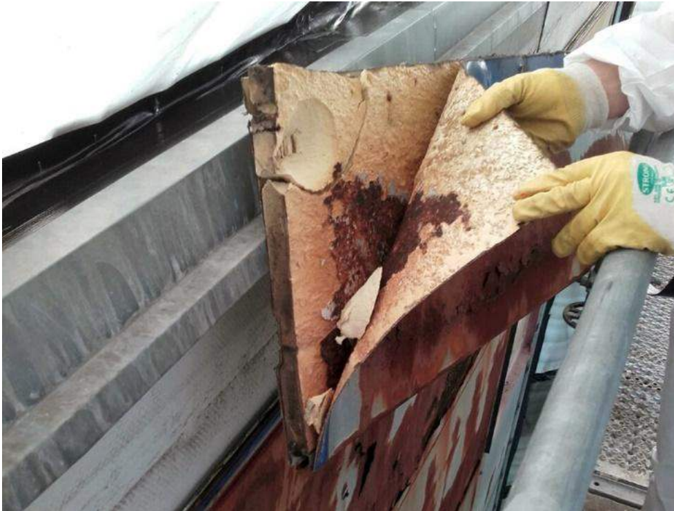
Figure 9. The rust of the façade panels was also in the inside layer, making the sheet metal detach from the PU foam core
